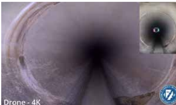
A high-resolution image of a sewer interceptor using drone technology.
