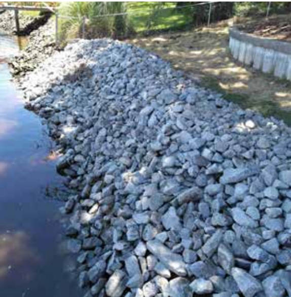
A completed retaining wall made from riprap
