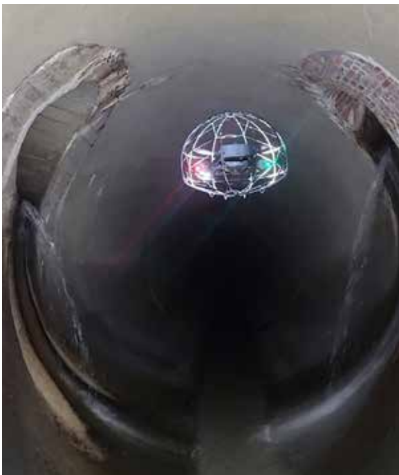
The drone being flown inside a sewer pipe in Macomb County.
