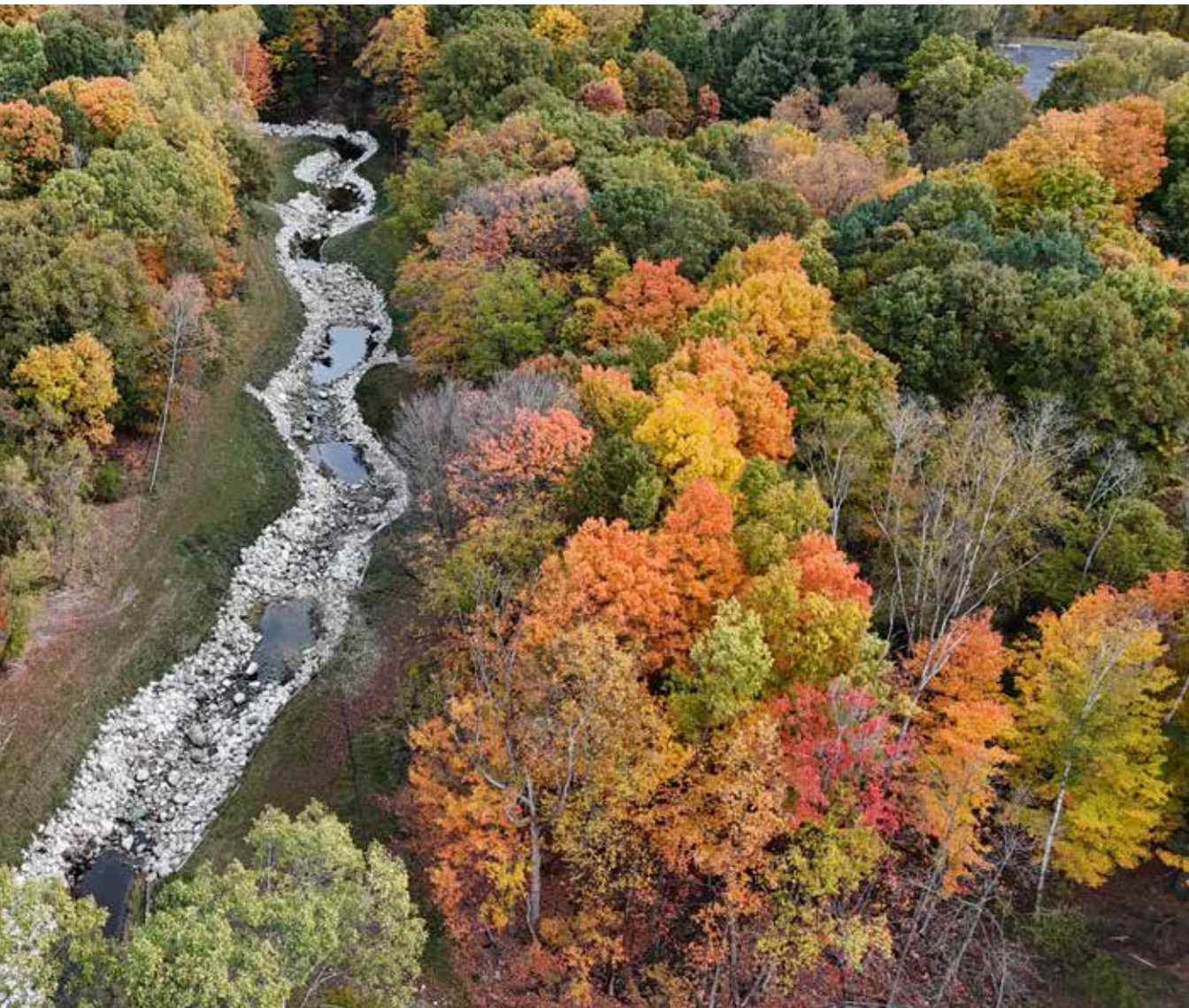
The Ives Drain in Mecosta County post construction
