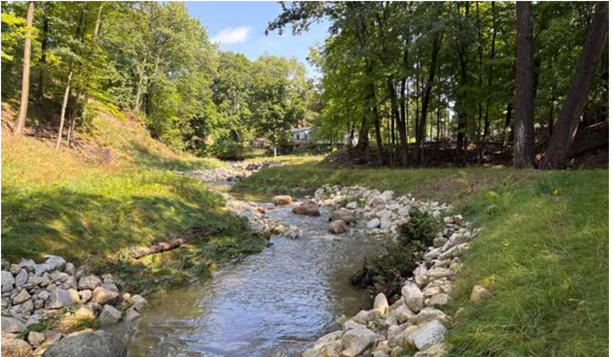
Restored Ives Drain after project completion
