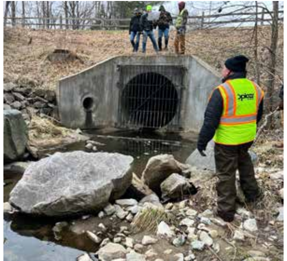
84-inch diameter storm sewer outlet along the Ives Drain
