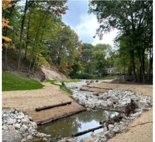
Finished drain after construction
