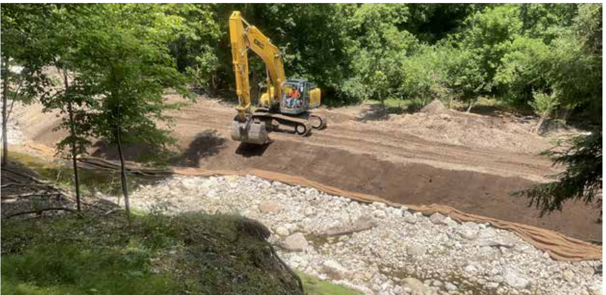
Crews performing slope stabilization during the project construction
