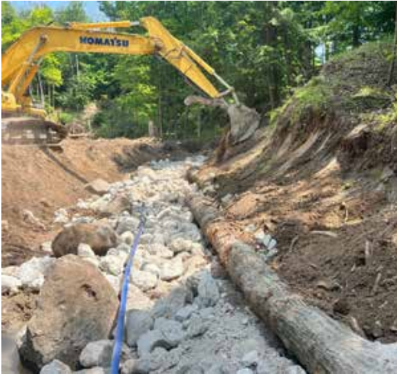
Bank stabilization and drain restoration under construction
