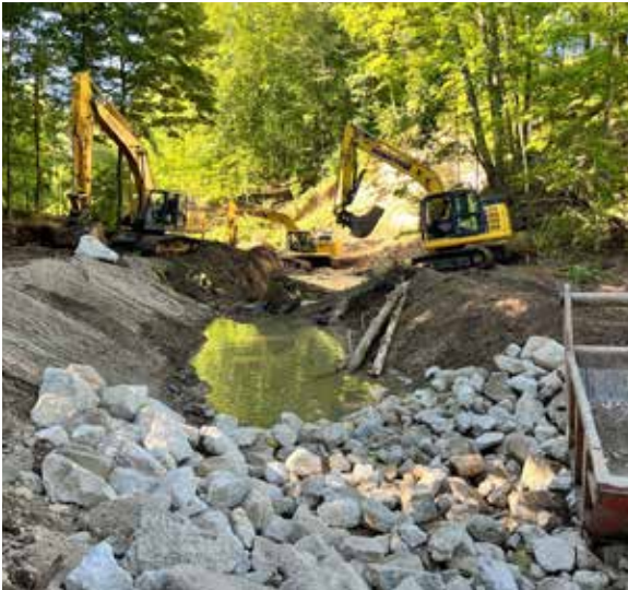
Drain restoration and bank stabilization under construction
