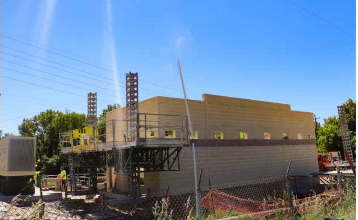
Construction of the Gage Drain Pump Station building.
