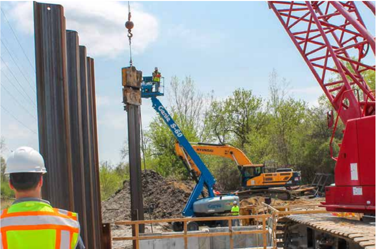
Spicer Group engineer overseeing the installation of sheet pile wall.
