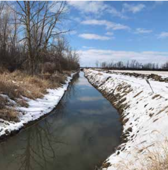
Winter time work on Gage Drain Open Channel Division.
