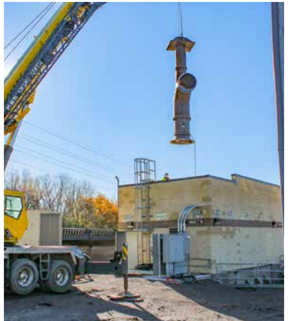
Installation of one of the new axial-flow pumps.
