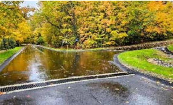
One of the trench drains across the roadway
