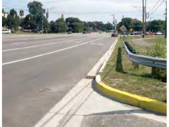
Sewer repairs completed, and Elizabeth Lake Road successfully re-opened to traffic.
