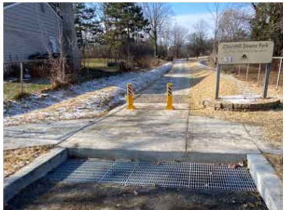
Restored park entrance where the outlet control structure is located.
