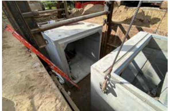
Setting the 10' x 12' box culvert sections of the outlet control structure.
