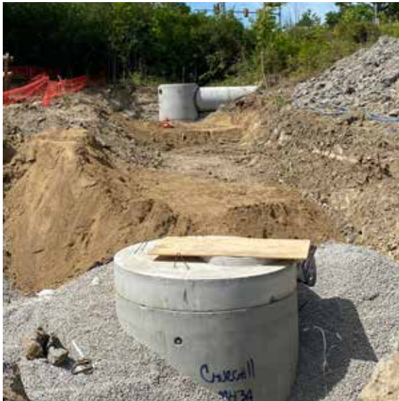
Storm sewer installation on the site north of the floodplain area.
