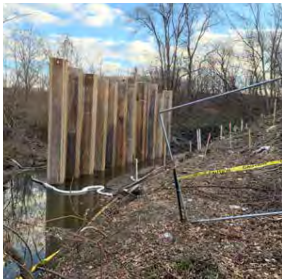
The complete steel sheeting that was part of the intensive effort to halt the flow of old diesel fuel that had leaked in the Bear Creek Drain, part of a $1 million cleanup.
