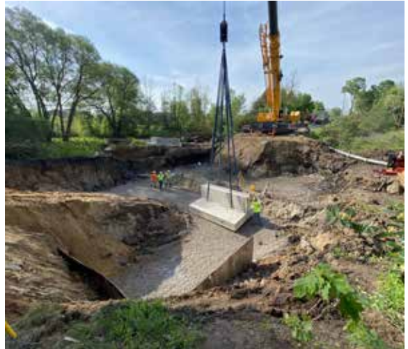
Installation of culvert crossing on the Little Tobacco River Intercounty Drain.
