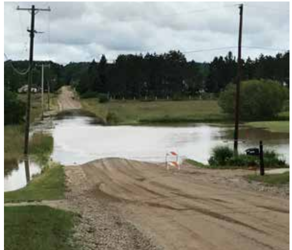
Dunlop Road flooding at the upper extent of the Little Tobacco River Intercounty drainage system before the improvement project.
