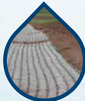
Tied Concrete Block Mat
