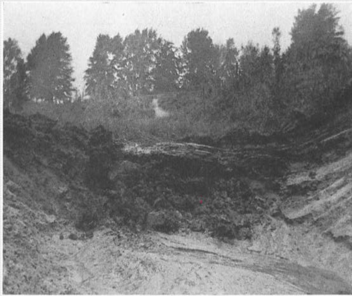
Starting place of the Ramey-Chandler Drain, affecting Ingham & Clinton counties, before construction.
