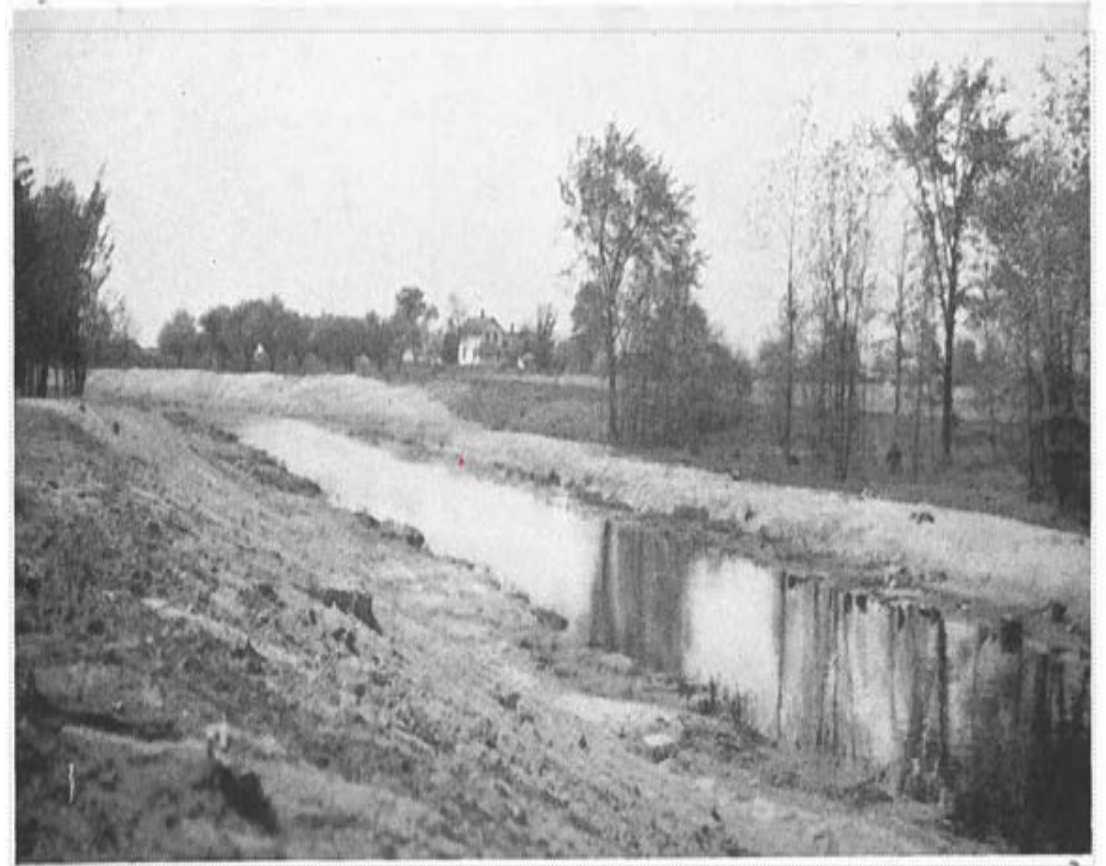
Looking Glass River Inter-county Drain in Clinton and Shiawassee Counties after construction.
