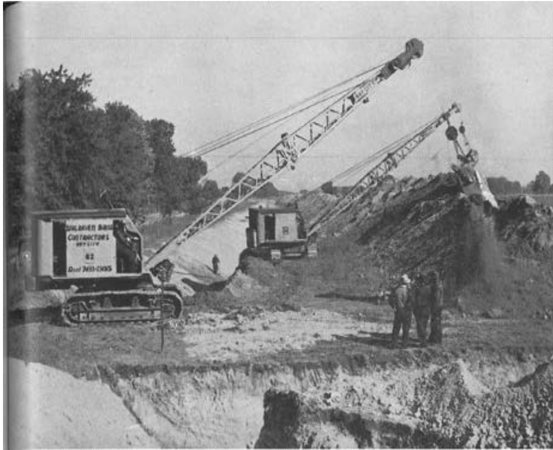
Construction of a 40 ft. width of bottom drain.
