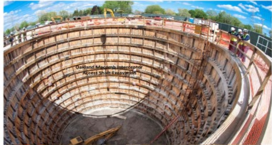
Oakland Macomb Interceptor Sewer 22 mile long, 12.5' Tunnel - 105' deep
