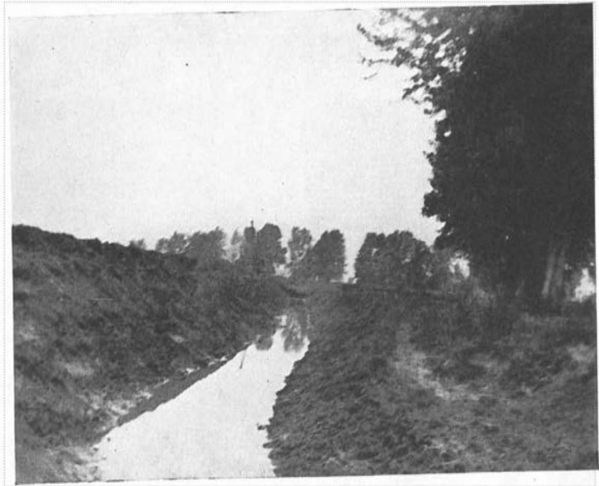
Finished portion of the Ramey-Chandler Drain, after construction.
