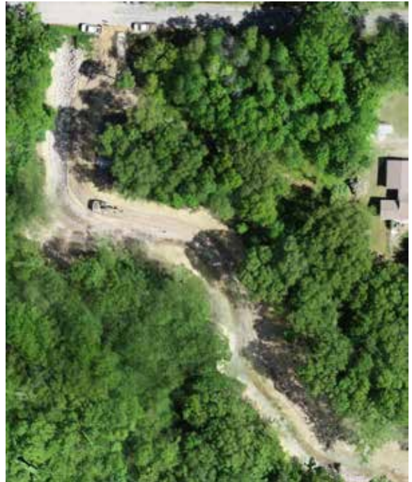
Buttermilk Creek, During Construction
