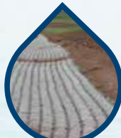
Tied Concrete Block Mat
