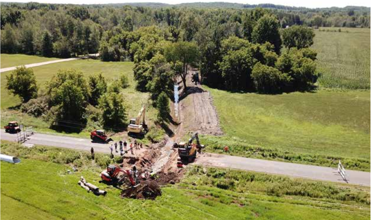
Aerial view of the drain and dig site.
