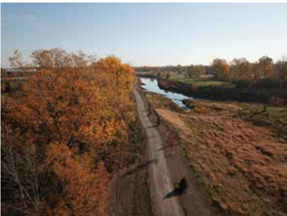
The completed hike/bike trail along the Sterling Relief Drain portion of the 1.35-mile path
