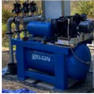
The airburst system gives a high-pressure burst of air through the microscopic intake screen to keep it clean from debris and vegetation.
