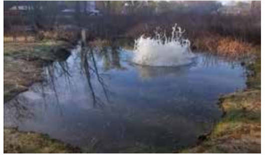
The airburst system gives a high-pressure burst of air through the microscopic intake screen to keep it clean from debris and vegetation.
