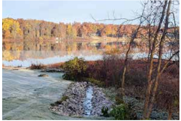
Photo showing the Drain’s outfall aeration channel as it outlets into the wetland system on the south end of Long Lake.
