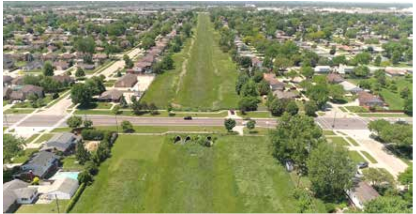
Aerial before construction
