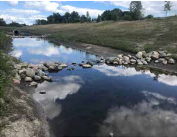
Check dam installed within the Sterling Relief Drain
