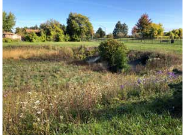
Updated and cleaned out culverts at Shoenherr Road
