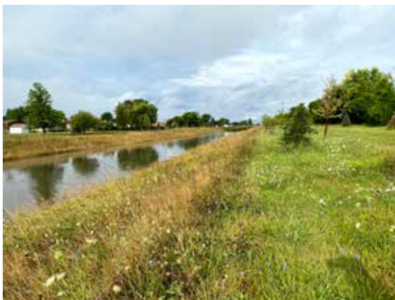
Drain corridor after construction
