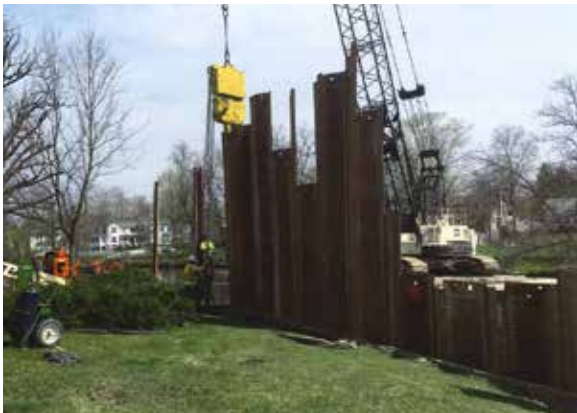
The rehabilitated southeast, northeast, and northwest quadrants of seawall include steel sheet piling and concrete caps.
