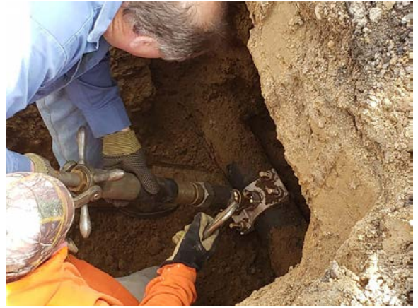
Contractor reinstating a service line connection
