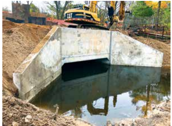
The photo above shows Lighthouse Creek Drain culvert before construction. The photo below shows the Lighthouse Creek Drain newly constructed box culvert
