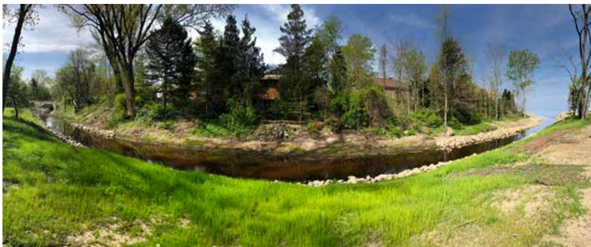
Restored Lighthouse Creek Drain outlet
