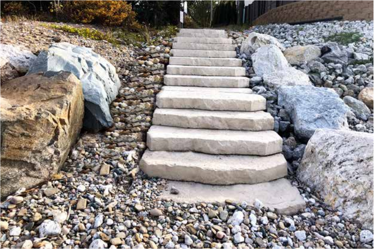
Stone steps were installed to accommodate public access to the beach
