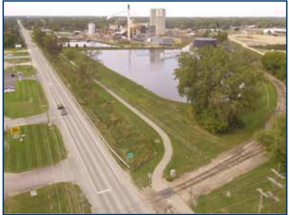
Croswell Drain Reach adjacent to M-90 Drone view looking west
