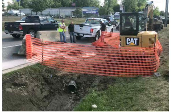
A pipe that allows a road ditch to drain in the Murdock-Ballard drain along Jefferson, south of Crocker, is seen.
