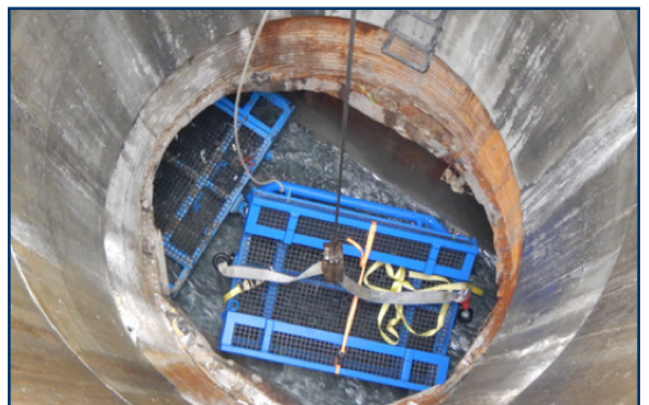
Work Sled Installation at Access Shafts
