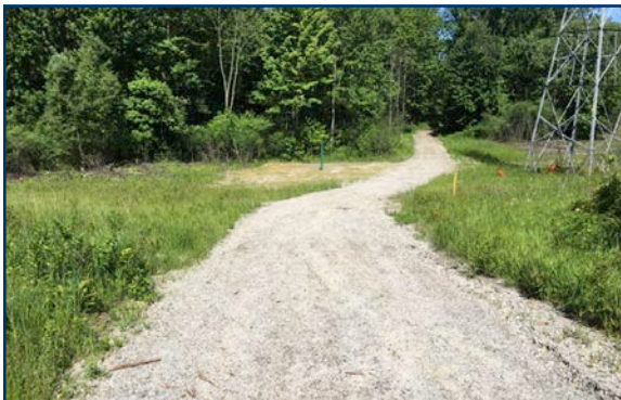
Site Restoration - Access Path in River Bends Park
