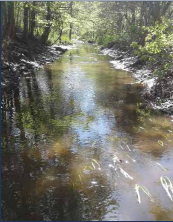
Figure 6: Debris Off Flood Plain
