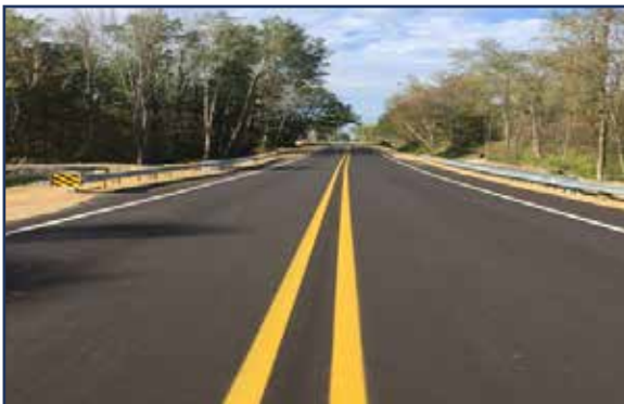
Paved finished product with culvert within restrictive right-of-way
