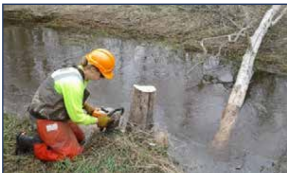
Figure 3: Clearing future obstructions to flow
