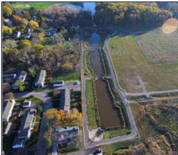
Photo looking south at the 3 Treatment Basins on the east side of the BWL property
