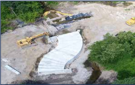
Aerial view of finished culvert
