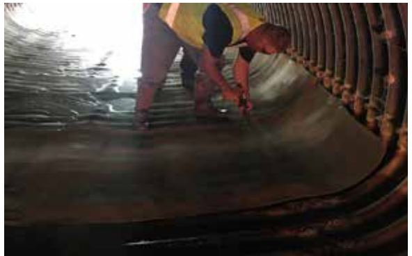
Securing CC8 panels with a Ramset tool and fasteners to invert
