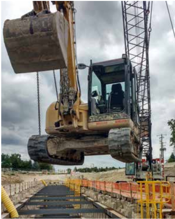
A mini-excavator is removed from the recovery shaft excavation site.
