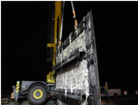
This screen, installed just upstream from the bypass pumps, illustrates the “ragging” associated with “flushable wipes” being disposed of in the sewer system. The wipes caused significant difficulties due to clogging up the pumping system.
