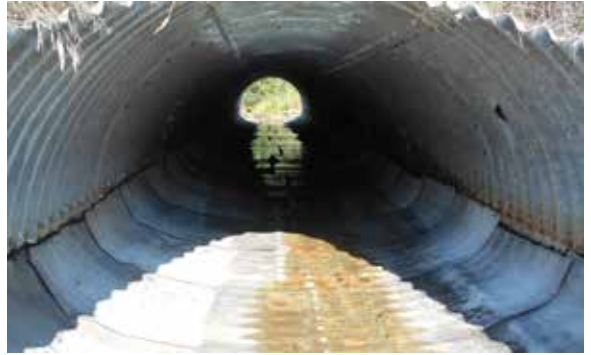
Completed CC8 invert rehab, with sealed edges
