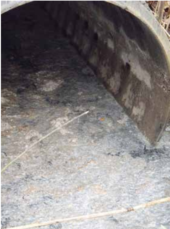
Gray scums downstream of an illicit connection. The E. coli concentration at this site was in the millions.
